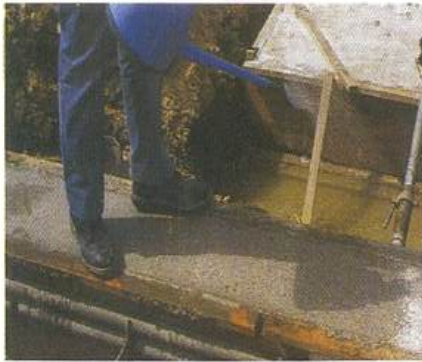
BRUSH OFF DIRT AND WET CONCRETE JOINT.
