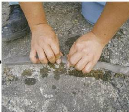
CONNECT TWO PIECES BY BUTT JOINT AT ENDS.
